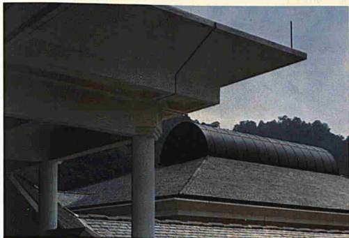
Eaves conceal the guttering of Kelab Darul Ehsan.
