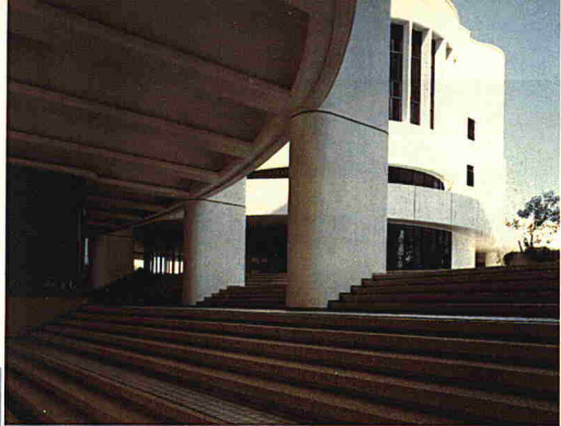
Adapting the principle of kampung architecture that frees the ground level for other uses.
